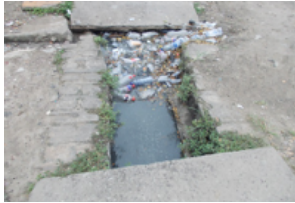
Waterway blockage (Kinshasa, February 2019)
