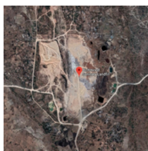
Richmond Sanitary Landfill (coordinates: S 20°05'00" E 28°32'00")
